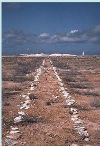
Remnants of guano tramway on Jarvis Island with guano stockpiles in the background. Source: Wikipedia
