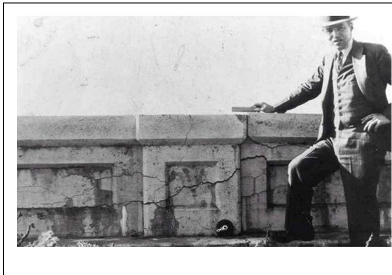
Figure 2.1: A typical ASR in concrete and Mr. Stanton (Stanton, 1941)
