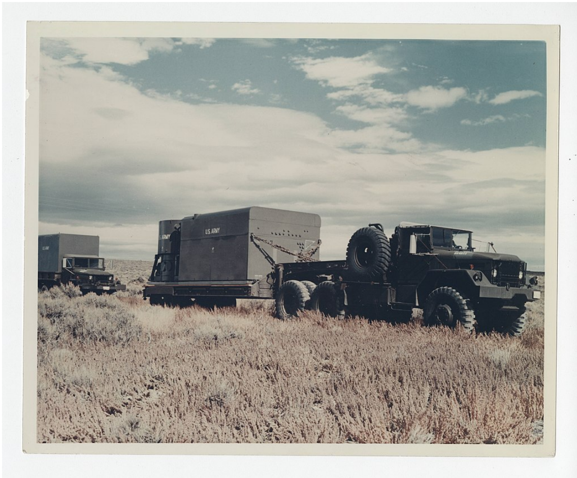
Figure 1.1: ML-1 Reactor Skid
