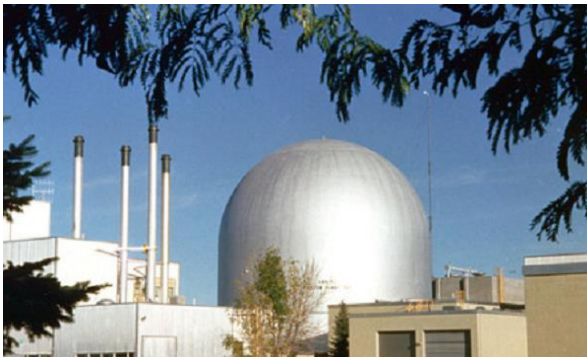
Figure 1.2. Experimental Breeder Reactor-II (center) with adjacent power plant (left) and Fuel Cycle Facility (right, which was later named the Fuel Conditioning Facility).
