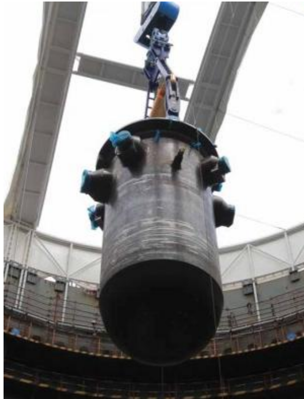
Figure 1.1: Reactor Pressure Vessel
