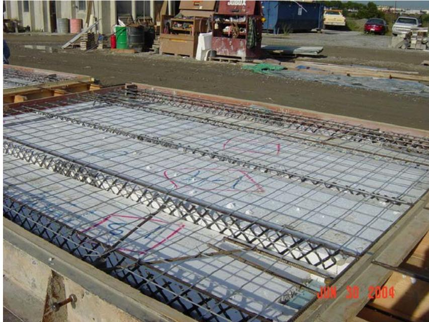
**Figure 14 – Composite Panel Production Prior to Pour**
