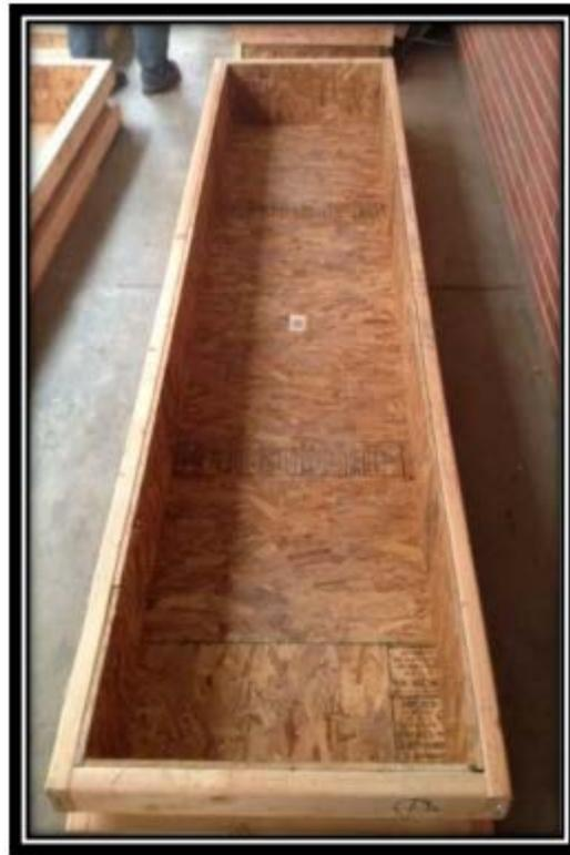
**Figure 40 – Wooden concrete form**
