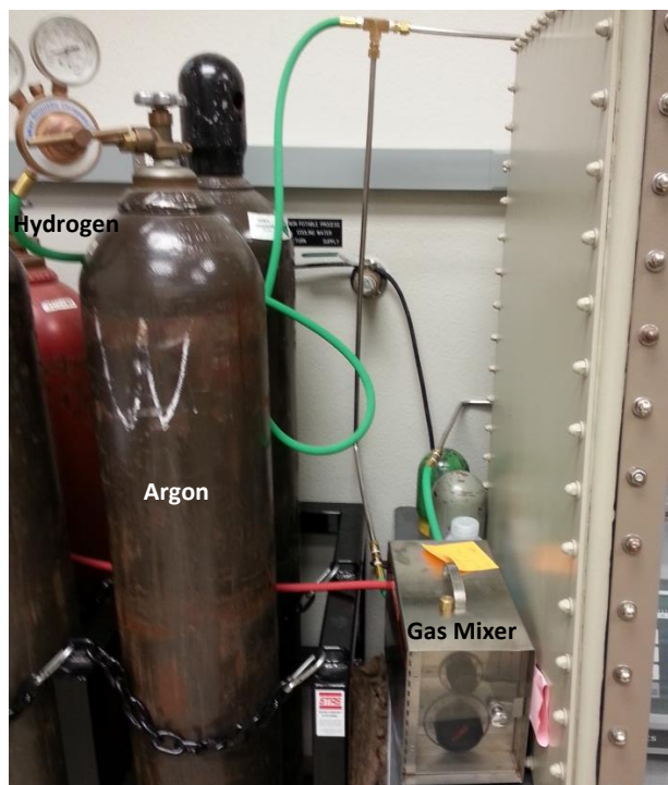
Figure 18 Detail of Gas Mixer
