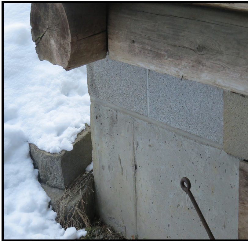
Figure 35: The divide between the original church and the added basement (Kleer-Larson 2016)
