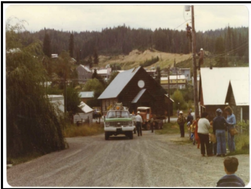
Figure 26: Workers disconnect power lines to allow Our Lady of the Woodland to pass through (Triplett 1980)
