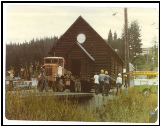
Figure 23: The bridge (Triplett 1980)
