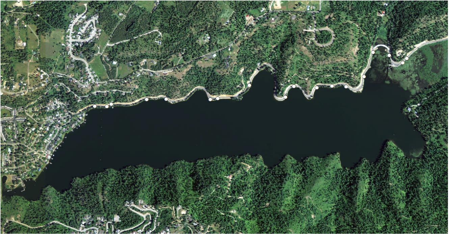
Figure I.2: Aerial image of Fernan Lake showing the locations of the culverts that run underneath Fernan Lake Road.
