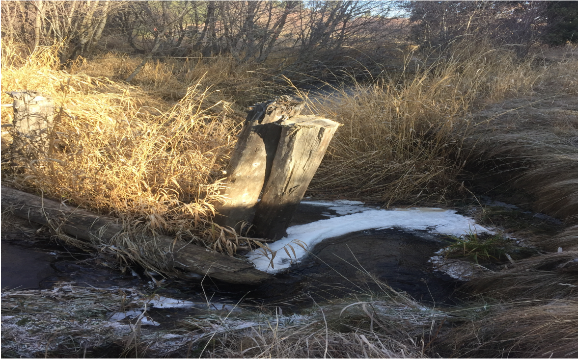
Image 4: Phase 2 Choke Structures
