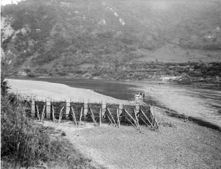
Figure 5.6, An old lamprey weir, picture and description cited from Te Ara “This utu piharau (lamprey weir) is on the banks of the Whanganui River, shown here in the late 1800s. Lamprey weirs were built around March, before winter rains swelled the river.”
