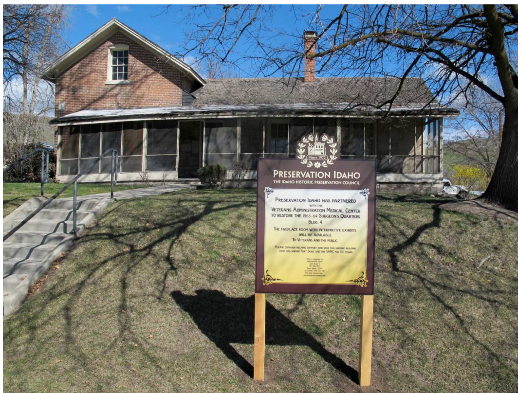
Figure 3.3. The Surgeons Quarters Prior to Excavation and Renovation, 2014.
