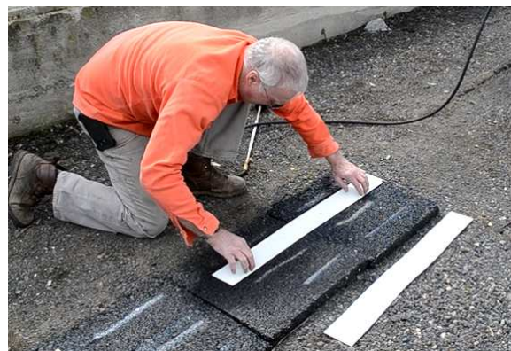
Placing the thermoplastic hot tape
