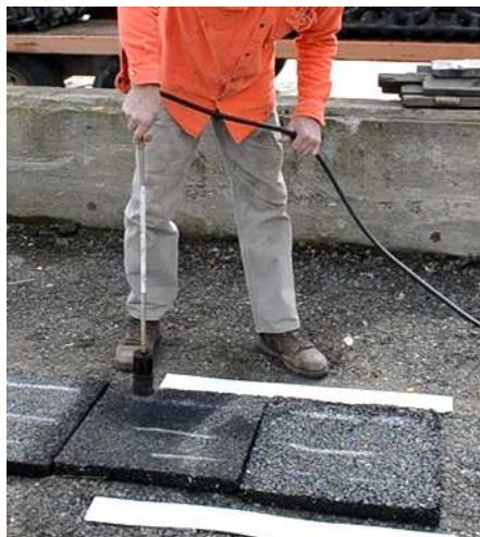
Preheating prior to application
