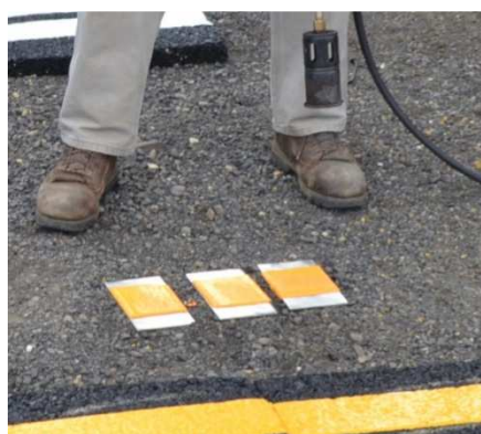
Applying thermoplastic markings on aluminum plates
