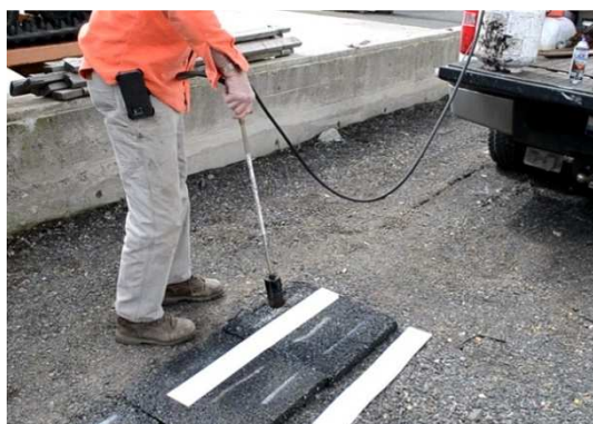
Heating up the thermoplastic tape
