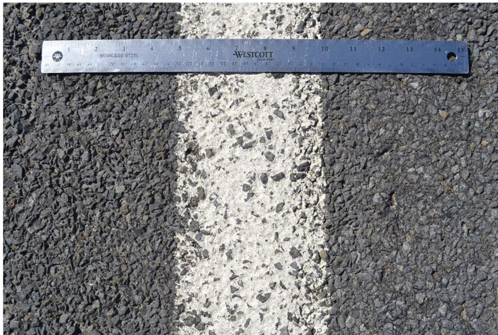
Figure 3.1. Edge line white painted pavement marking
