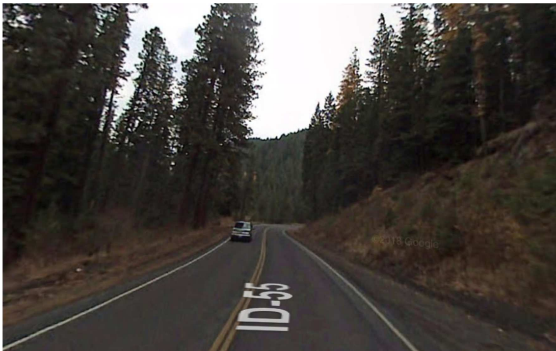
Figure 1.2. Road with a good pavement marking condition.
