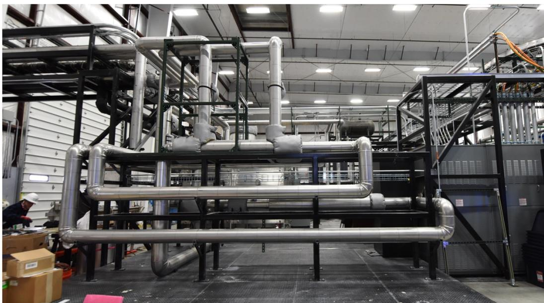
Figure 6-1. Photo of MAGNET Piping at the Completion of Construction
