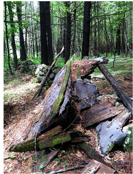
2.2 Stone Wall in Clough Park
