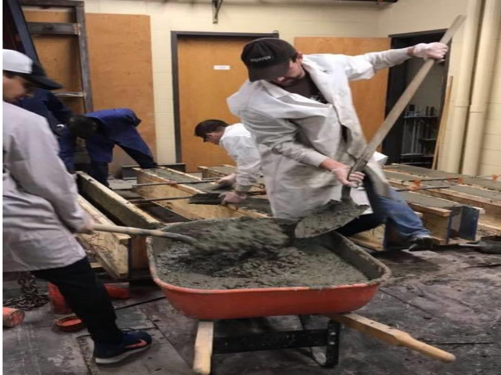
Figure 4.15: Pouring concrete into formwork
