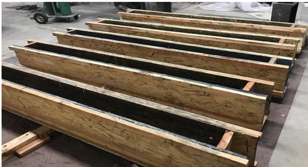
Figure 4.1: Prepared wooden formwork for concrete beams
