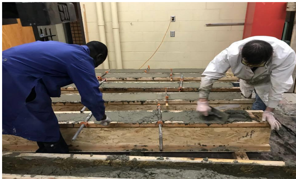
Figure 4.16: Leveling surface of concrete
