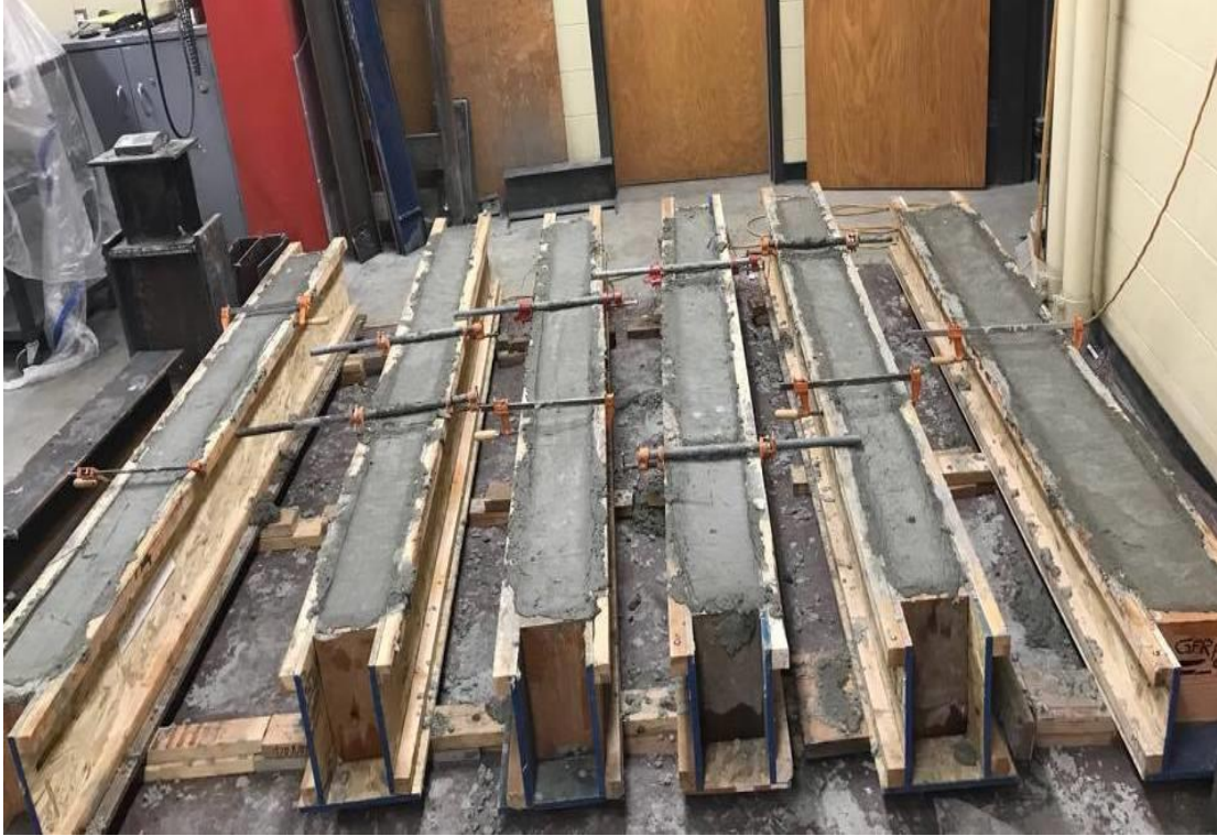
Figure 4.17: Casted concrete beams with clamps
