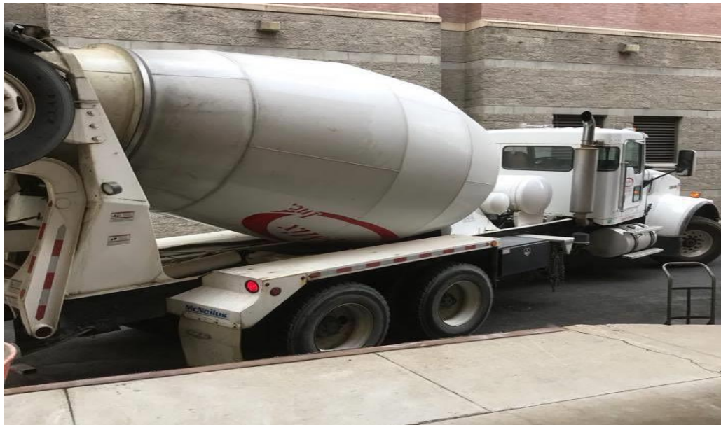
Figure 4.14: Premix concrete truck
