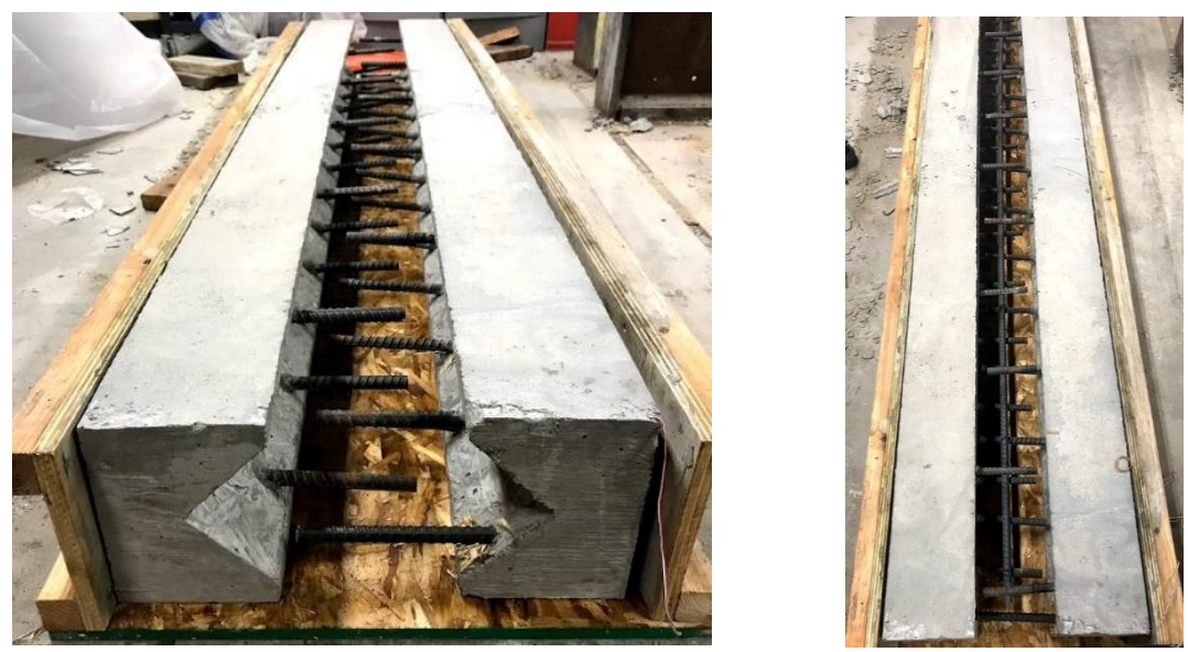
Figure 2.13 Form work for UHPC connection
