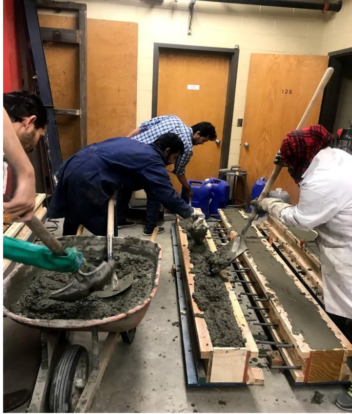
Figure 2.10 Casting of precast panels
