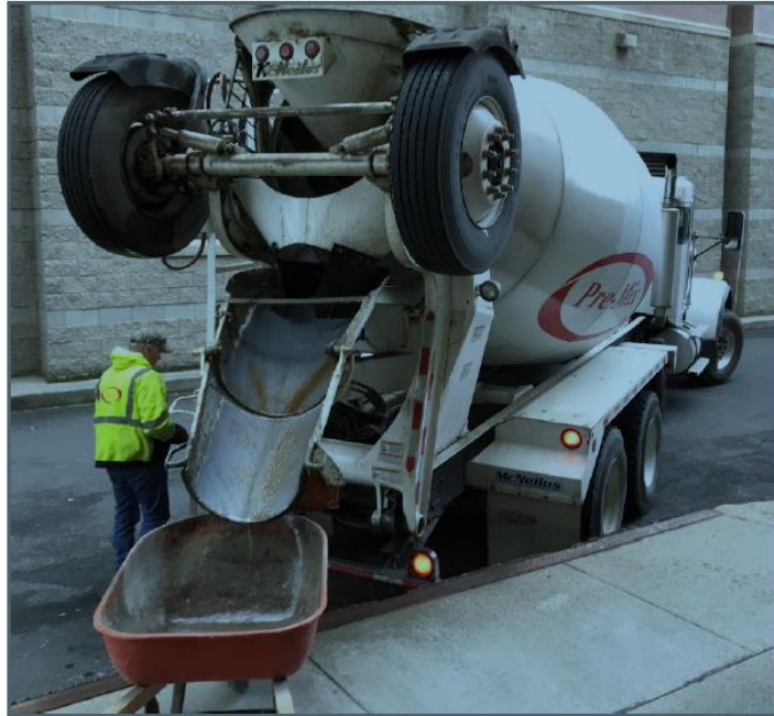
Figure 2.8. Pre-Mix Concrete Plant unloading HSC from their truck outside BEL
