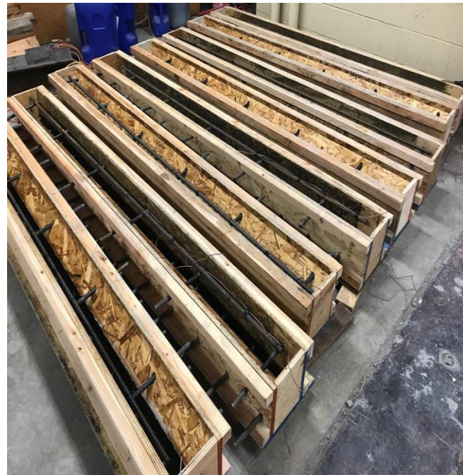
Figure 2.9. Wooden forms before pouring concrete
