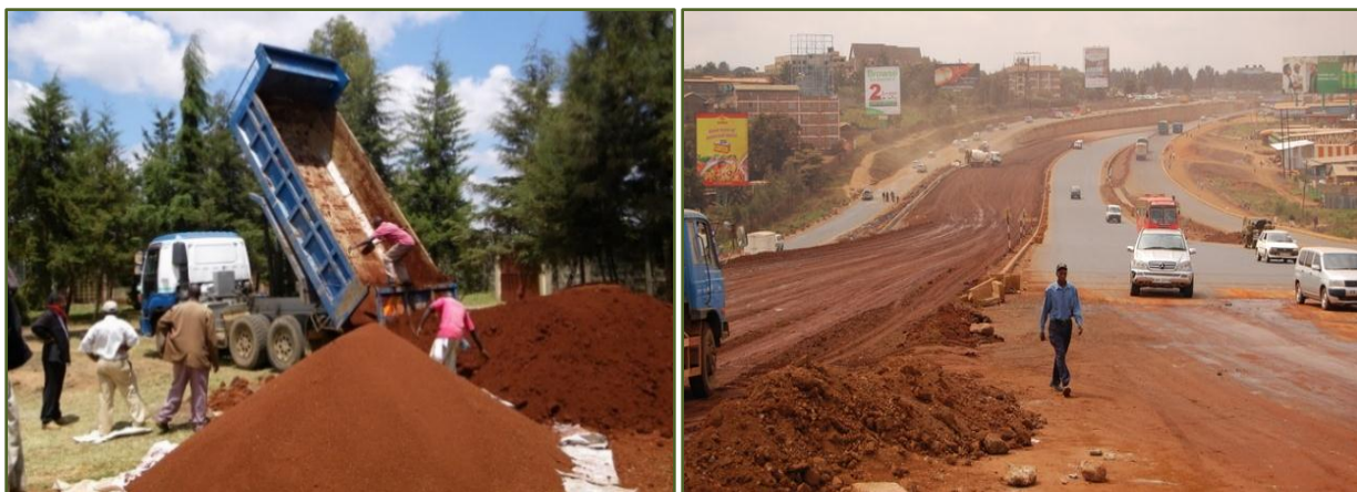
Photo 2: Red volcanic soil used in greenhouse farms and building tarmac road
