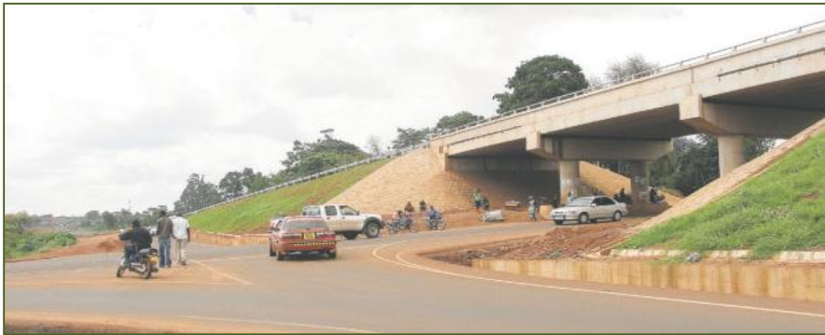
Photo 10: A section of the 25-km Northern Bypass in Nairobi
