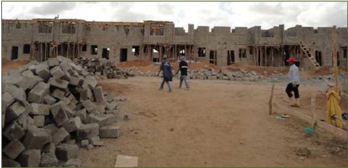
Photo 4: Constructions using artisanal dimension stone in Nairobi
