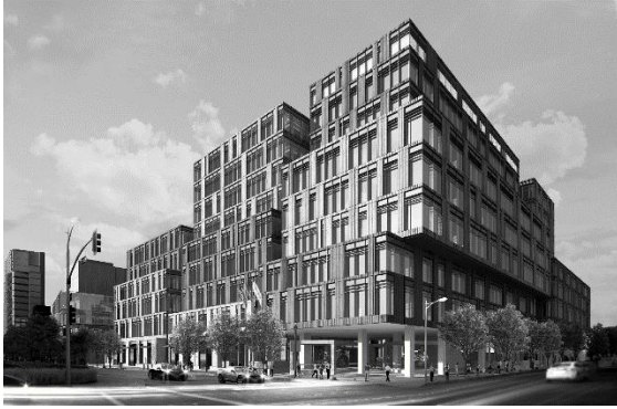
Figure 3-1: Case Study Building
