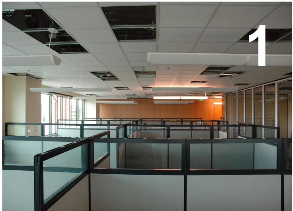
Figure C1: Space #01- Boise, ID – Open office space – 8 th floor
