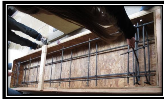
Figure 16: Solid Slab Reinforcement
