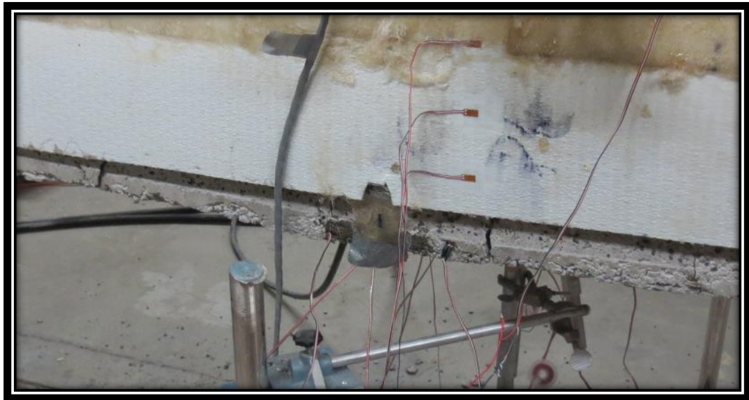
Figure 123: Full Scale 10" FPCS Cracking
