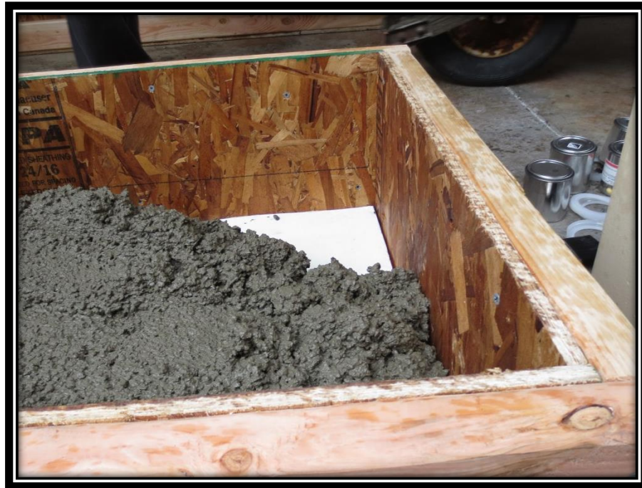
Figure 58: Concrete Poured on FRP w/Adhesive (Wet Bond)
