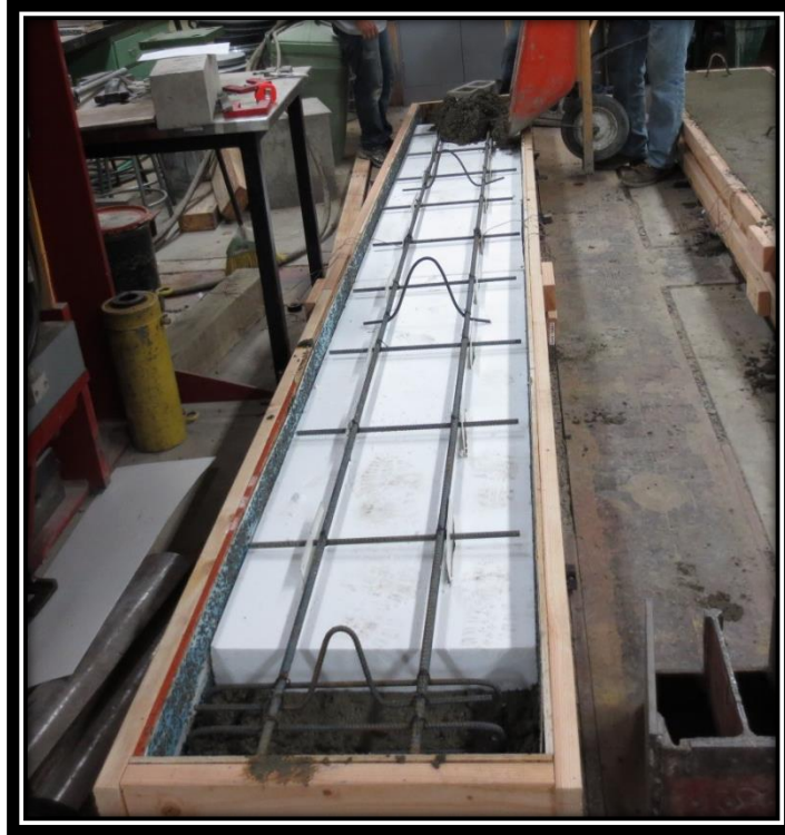
Figure 107: Insulation Installation
