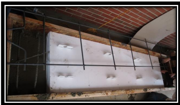
Figure 11: 6'' Discrete Shear Connector Slab Fabrication
