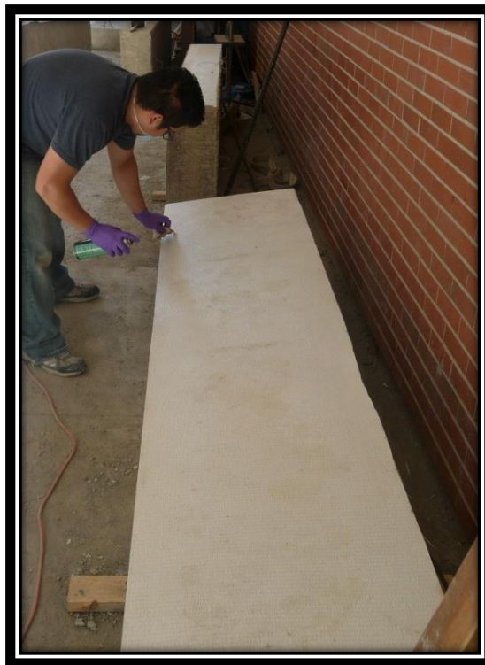
Figure 82: Abraded Surface Cleaning
