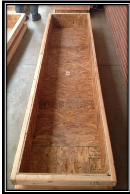
Figure 7: Wooden Concrete Form
