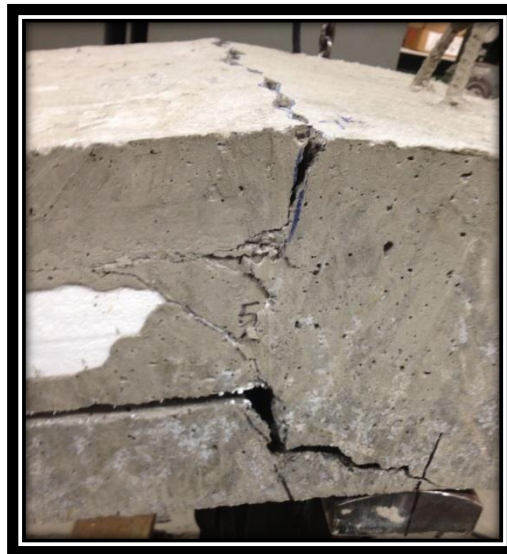
Figure 43: Shear Failure (Profile View)
