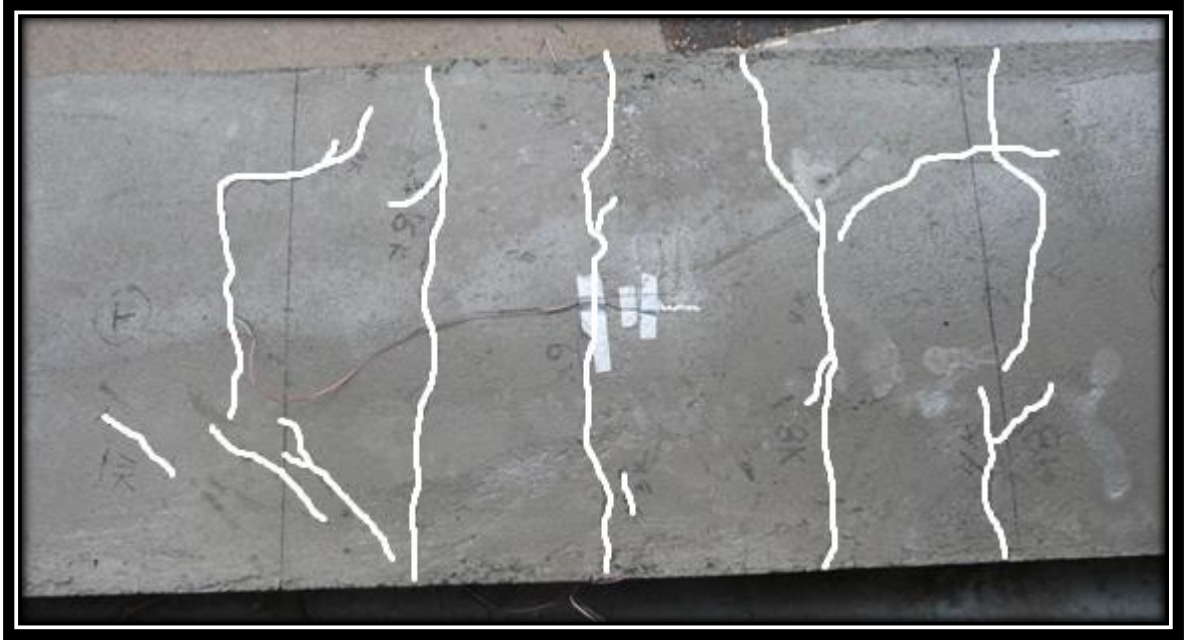
Figure 72: Continuous FPCS Specimen 1—Crack Pattern (Bottom of Specimen)
