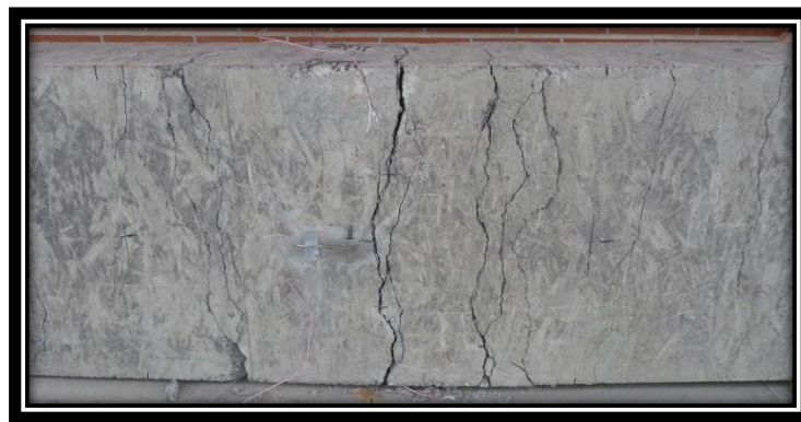
Figure 44: Bending Failure (Bottom of Specimen)
