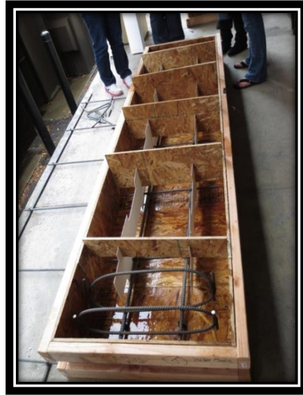
Figure 15: Continuous Connectors
