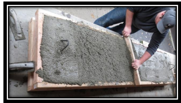
Figure 12: 6'' Discrete Connector Slab Finishing
