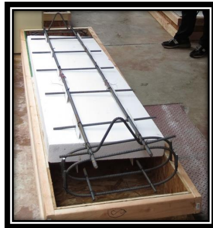
Figure 14: Cage, Insulation, and Shear Connectors
