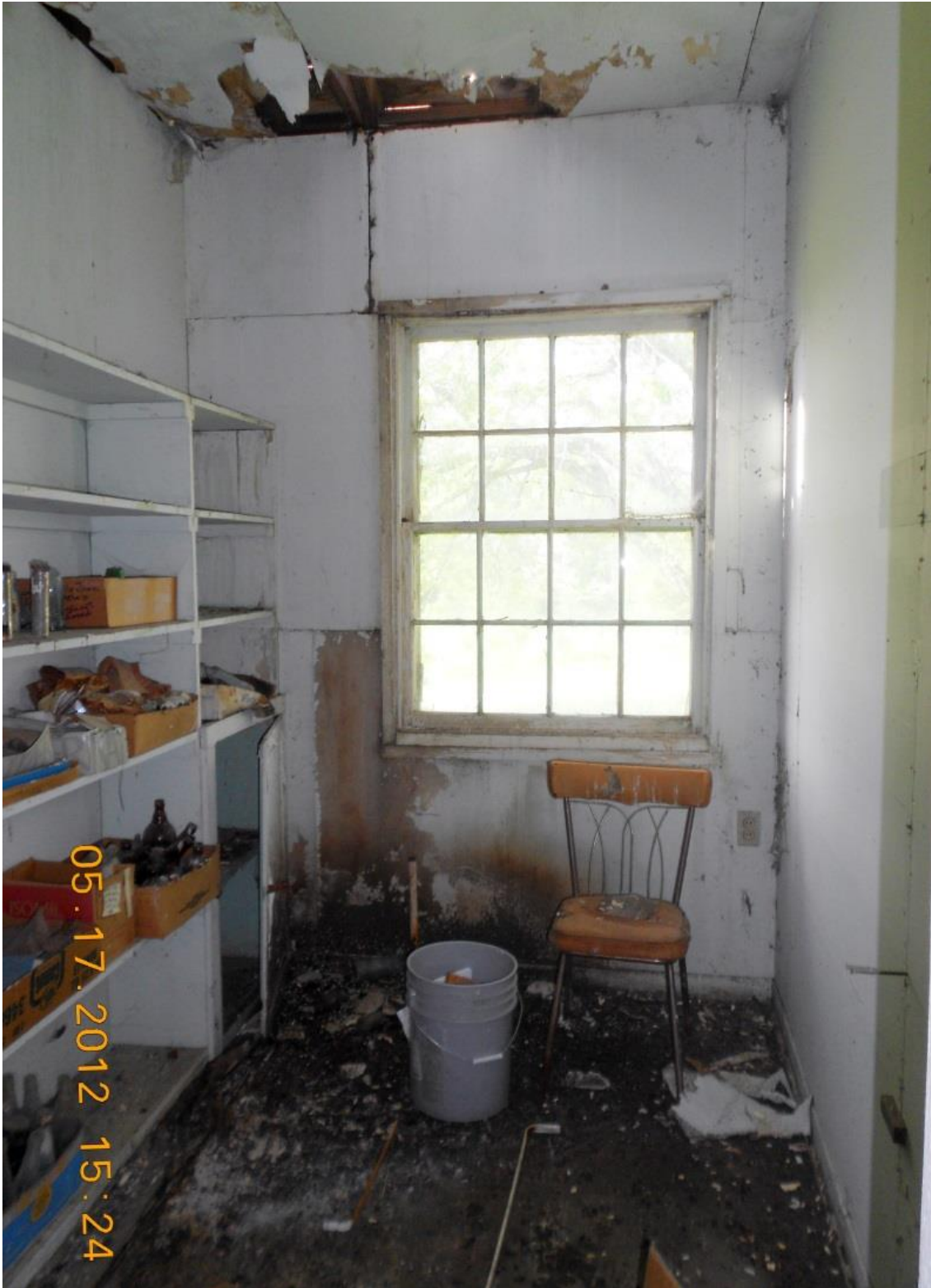
FIGURE 5. Room inside T8. (Photo by author, 2012.)
