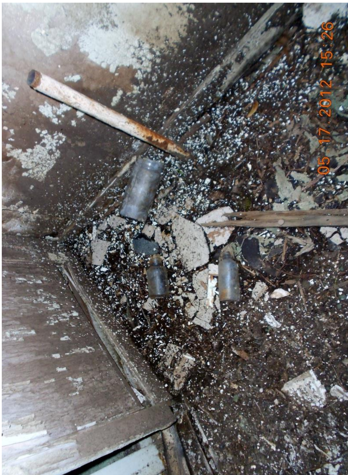
FIGURE 3. Room inside T8. (Photo by author, 2012.)
