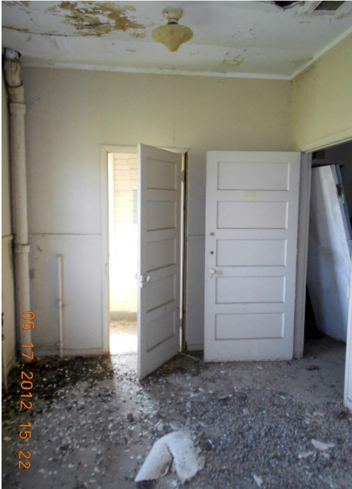
FIGURE 4. Room inside T8. (Photo by author, 2012.)
