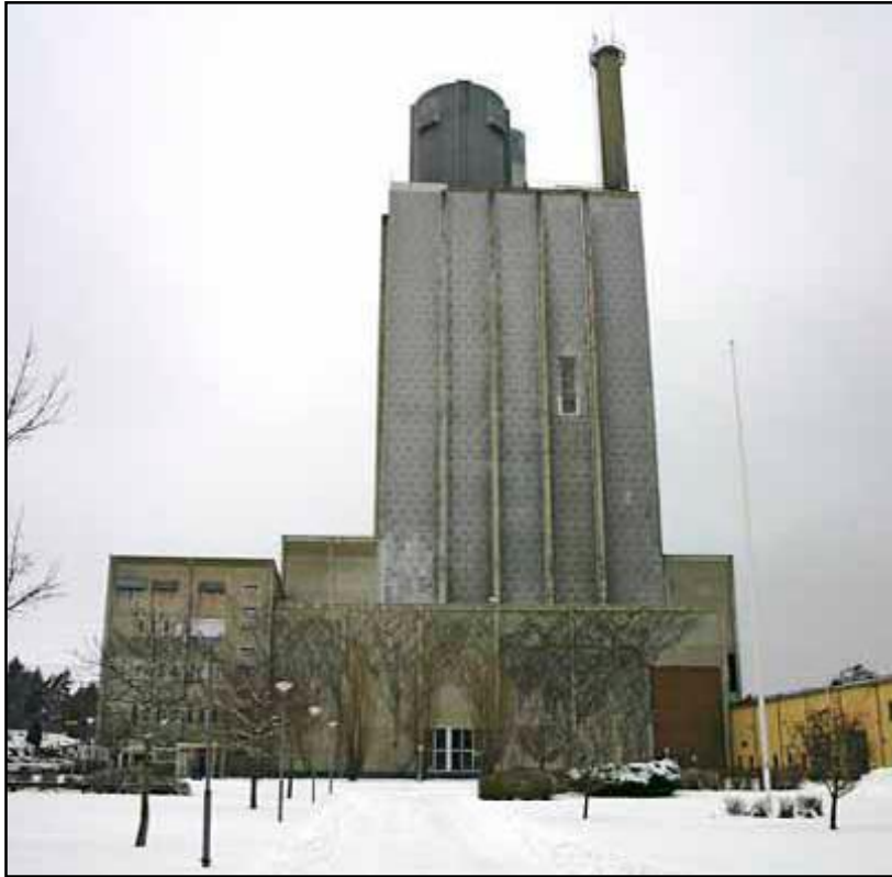
Figure 2-2: External view of the full-scale R4 Marviken Power Plant
