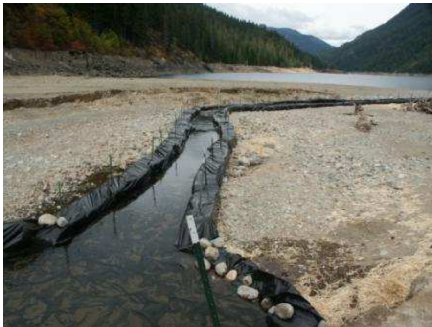
Figure 1.2. Passage channel created in the varial zone of Kachees Reservoir, Washington.
