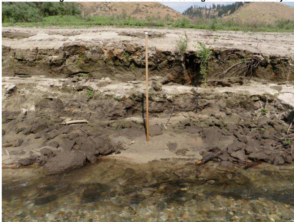
Figure 2.6. Example of unstable bank in the varial zone of the MFBR, Arrowrock Reservoir. Other sections of bank were actively sloughing off, but unsafe to photograph. A 2 m long stadia rod is in center of the photo for scale.
