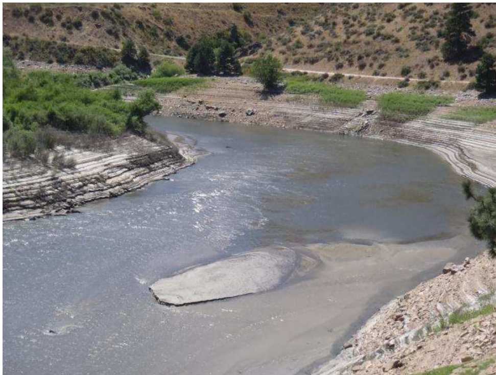
Figure 2.19. Relatively short and narrow delta in the varial zone of the MFBR Arrowrock Reservoir. This photo was taken at a relatively high water level (966.7 m asl) on July 31, 2012.
