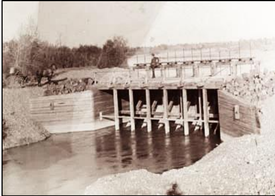
Figure 1.9: Main Canal Gate completion.
