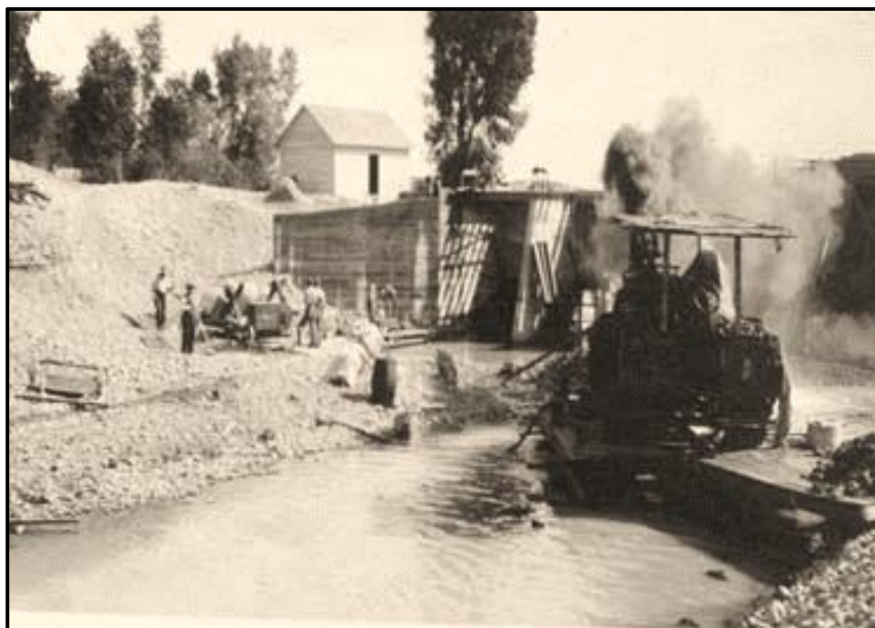
Figure 1.8: Main Canal Gate construction.
