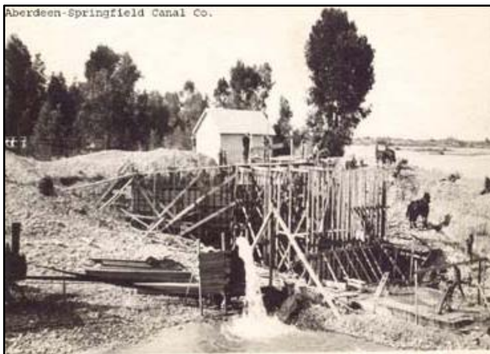
Figure 1.7: Beginning construction of the Main Canal Gate.
