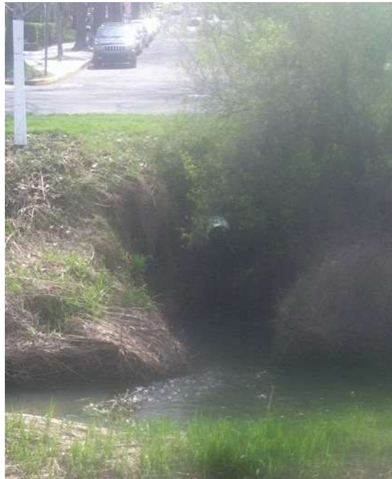
FIGURE 4.16 Evidence of localized scour capacity of stormwater outfall in urban reach of Paradise Creek.
