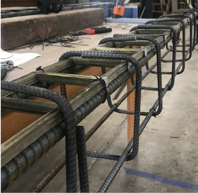
Figure 3-5: 5 GF/ST Hybrid Reinforcement Cage Close-up
