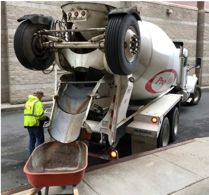
Figure 3-8: Pre-Mix Concrete Plant unloading HSC from their truck outside BEL
