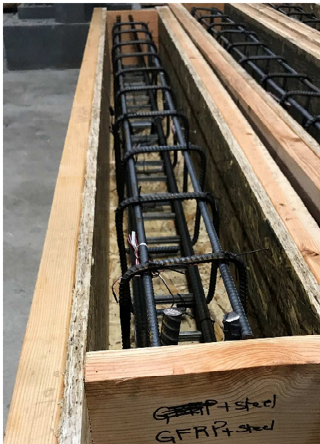
Figure 3-7: Installation of Strain Gauges and Reinforcement Cage for 5 GF/ST Beam
