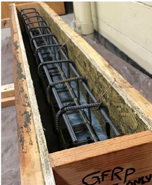
Figure 3-3: Installation of Strain Gauges and Reinforcement Cage for 3 GF Beam
