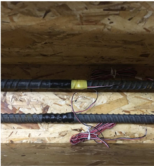
Figure 3-13: Strain Gauge Installed on the Steel Reinforcement
