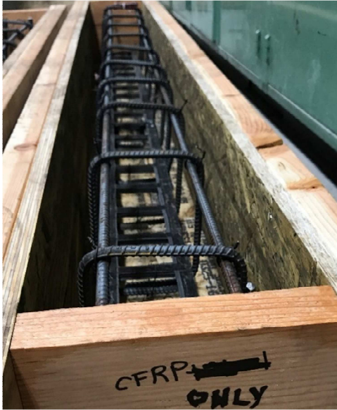
Figure 3-2: Installation of Reinforcement Cage for 2 CF Beam
