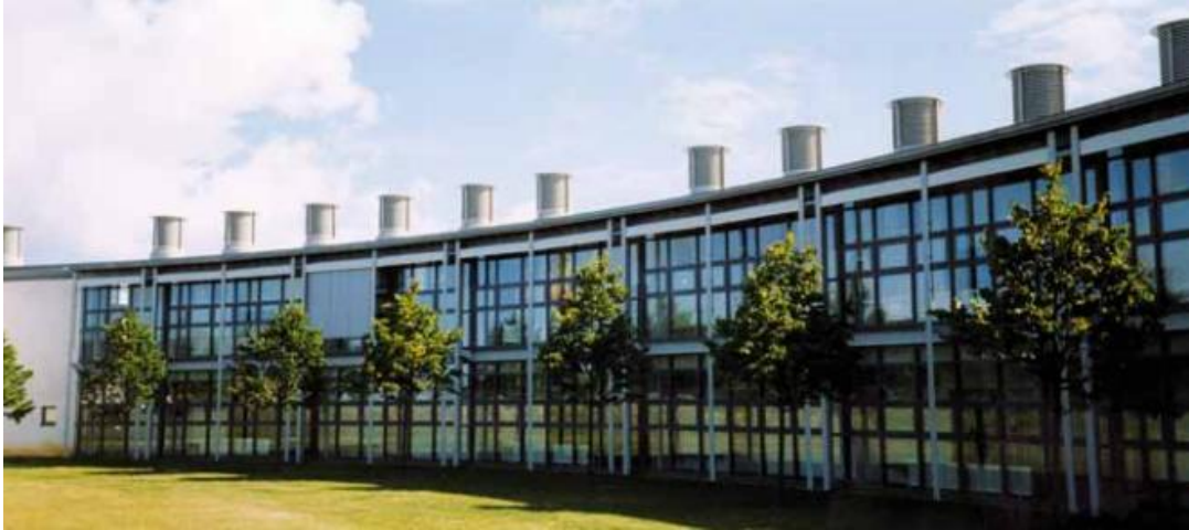
Figure 3-36: St Annes School in Haute Valley, Jersey [84]
