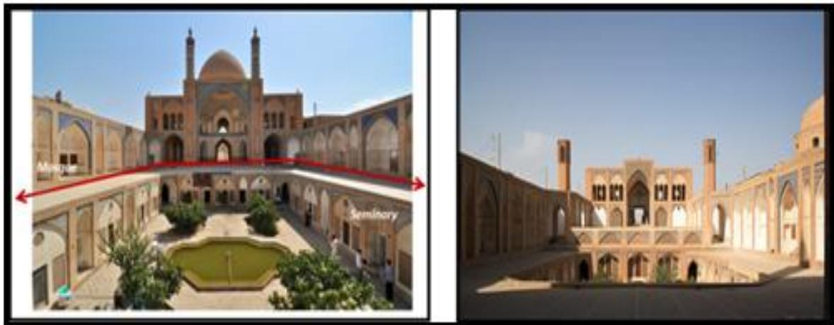
Figure 3-24: Seminary, Mosque, and Courtyard of Agha Bozorg Mosque Complex (Photo [74]) (Left), Wind Catchers at Northern Sector [72] (Right)
