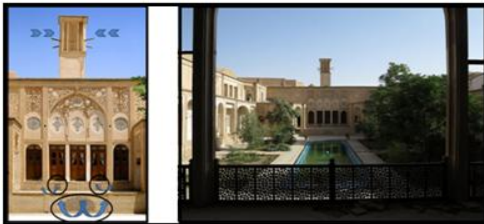
Figure 3-22: ventilation of Cellars under Winter- Living Quarter (Photo [70]) (Left), Winter-Living Quarter [70](Right)
