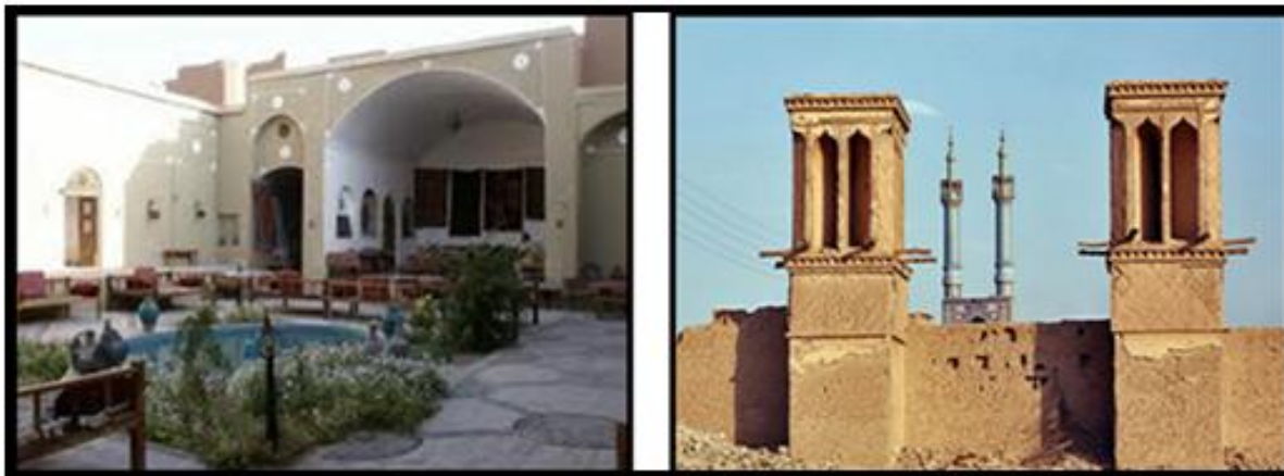
Figure 3-16: Courtyard in a Typical House, Tabas, Iran [67](Left), Wind Catchers on top of Summer Living Quarter [63] (Right)
