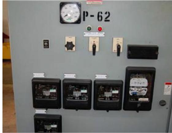
Figure 3.4 – Typical Feeder Protection Relay Front Panel
