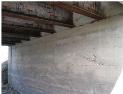
Figure 3.1: Representative steel girder bridge.
