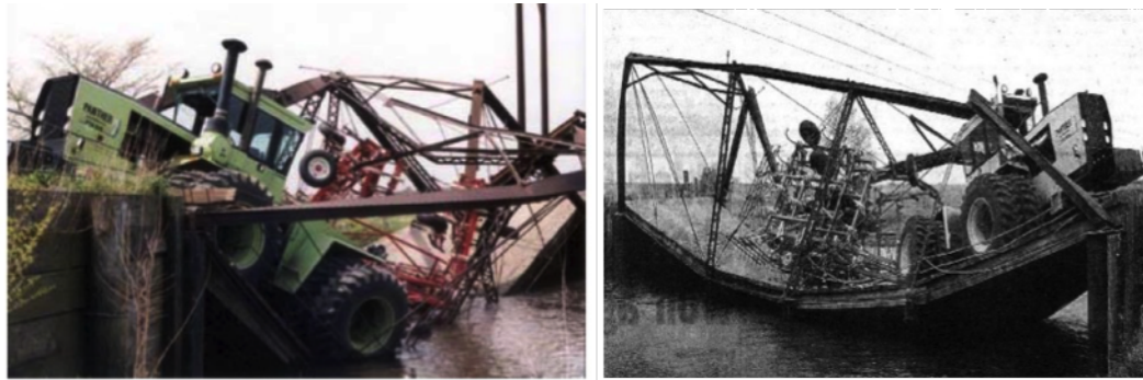
Figure 2.1: Bridge failures initiated by agricultural vehicles. [11]
