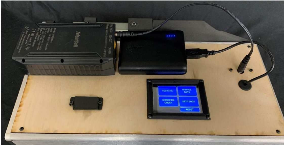
Figure 2.69 Batteries attached to case using hook and loop tape and plugged in.
