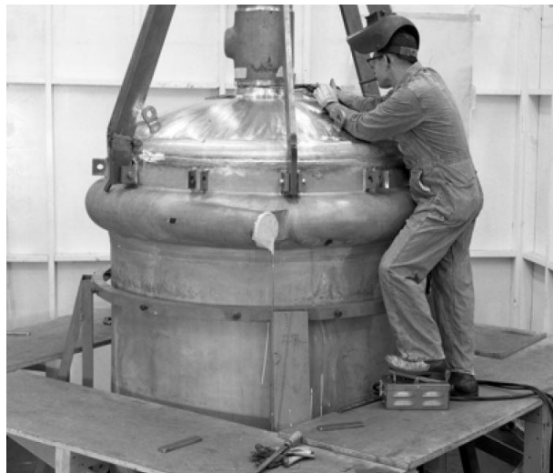
Figure 1-7 – MSRE Reactor Vessel Fabrication
