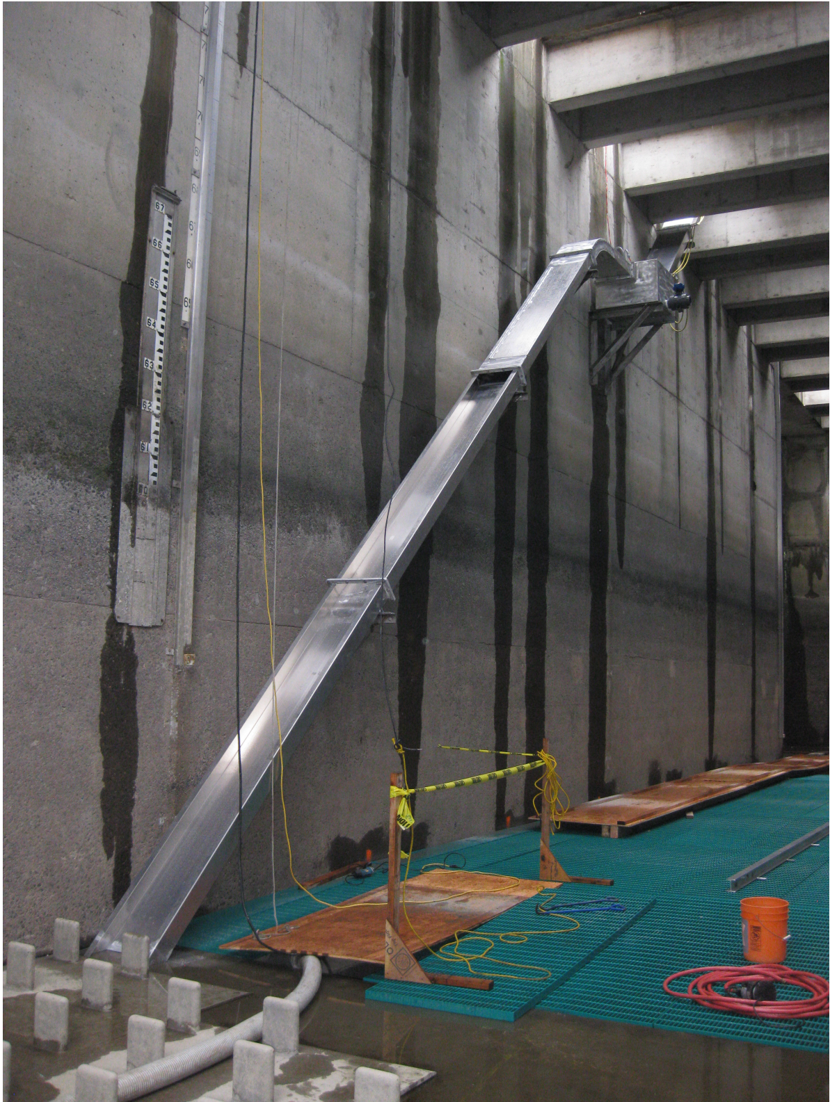
Figure 108: Completed LPS Structure
