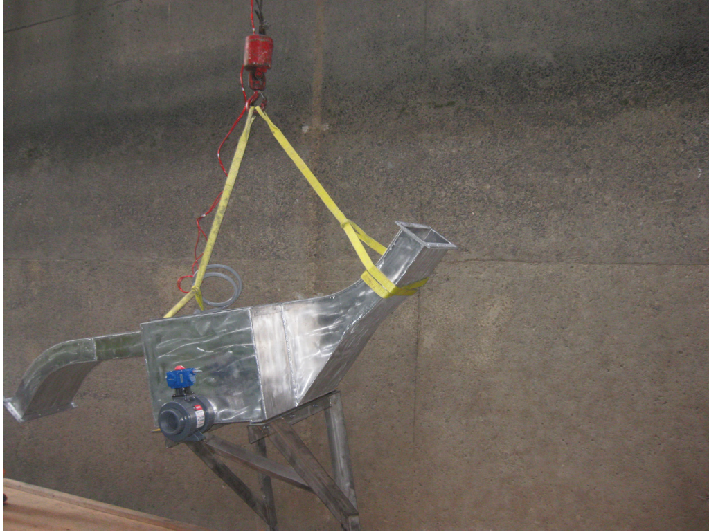
Figure 105: Lifting Rest Box into Place
