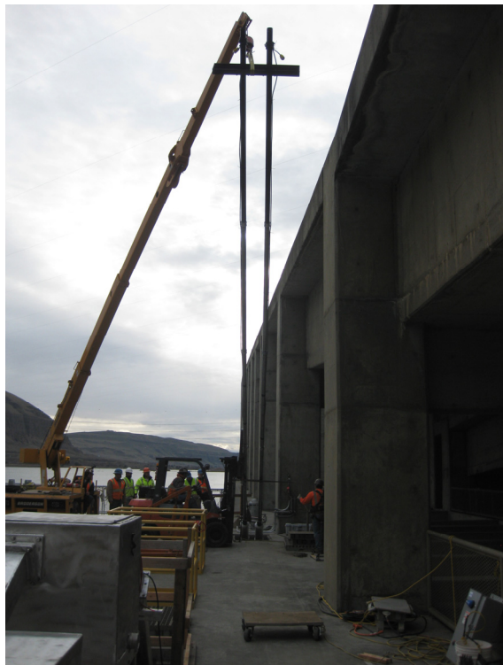
Figure 106: Lifting Pumps into Place
