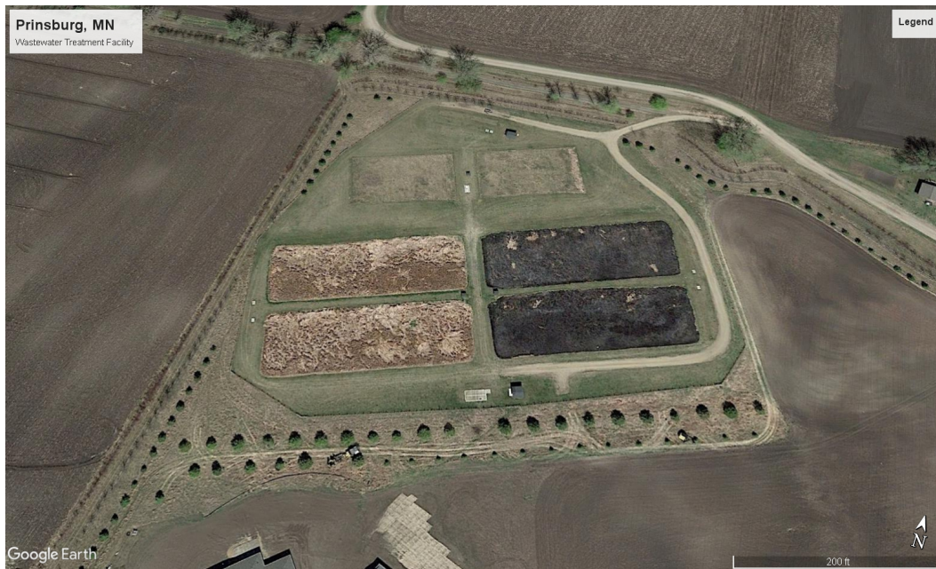
Figure 15. Aerial image of Prinsburg, Minnesota's wastewater treatment wetlands for a population of 497 (Google Earth, 2018).
