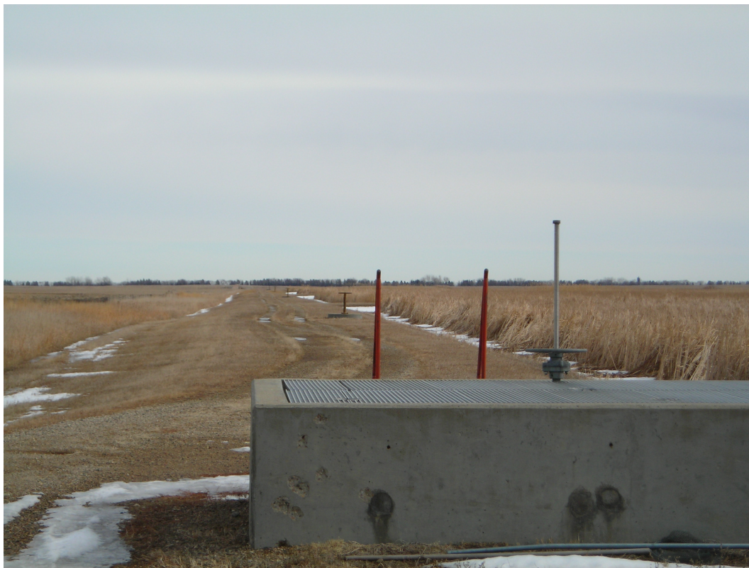
Figure 19. Photo of Minot wetland cells, courtesy of North Dakota Department of Health.
