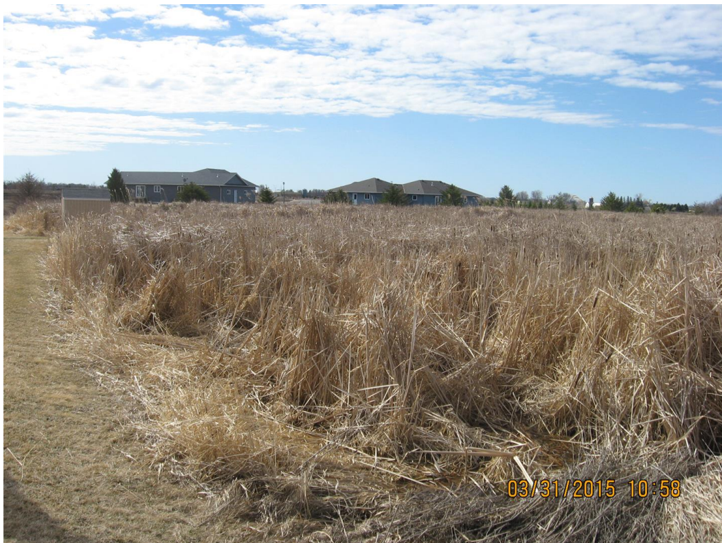
Figure 16. View of a wetland treatment cell, Prinsburg, MN. City of Prinsburg, 2015.
