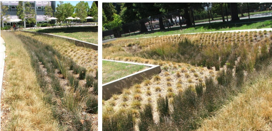
Figure 1.7-1.8 Stormwater Retention: Bio-swales in the landscape design retain surface water on site; Vanhoozer 2012
