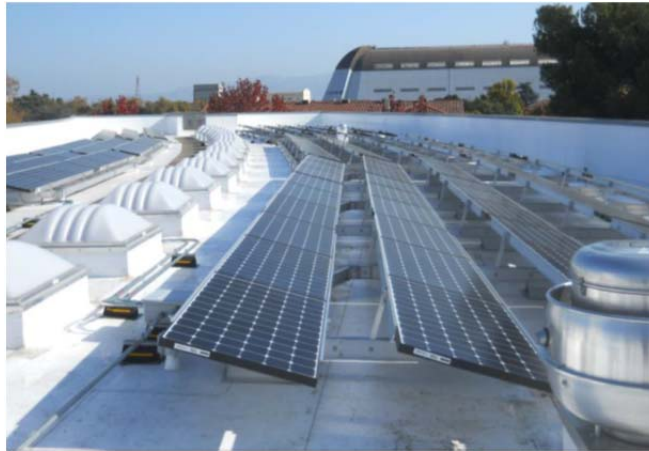
Figure 1.4 Solar Panels: Sunpower photo-voltaics on the roof generate about 30% of Sustainability Base's electricity; Schuler et al. 2010
