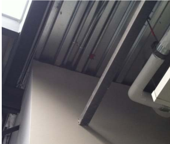
Figure 1.32 Mind the Gap: Gap between wall and corrugate ceiling generates sound excess in private spaces; Vanhoozer 2013
