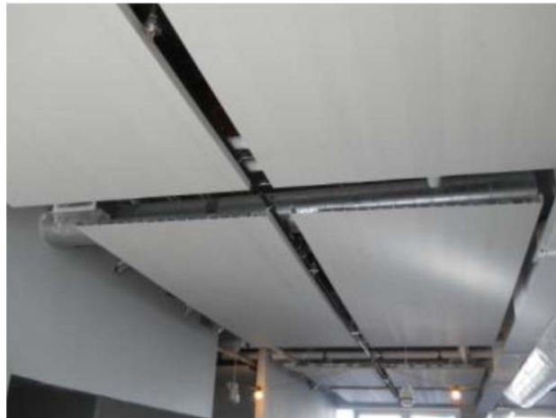
Figure 1.10 Radiant Cold: Radiant chill panels suspended from the ceiling provide cooling in summer months; Poll 2010
