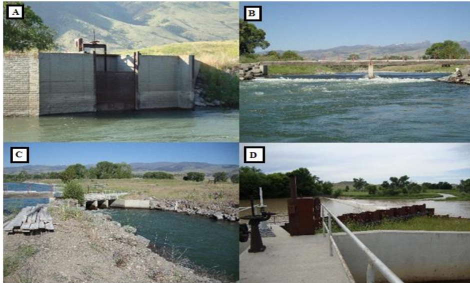
Figure 3.17 Examples of diversion types in the Yellowstone River Basin (A. Headgate without diversion; B. Side channel diversion; C. Multiple headgate partial channel diversion; D. Entire channel diversion with multiple headgates).
