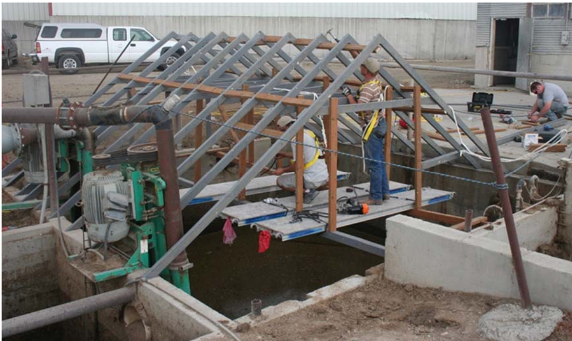
Picture 4. 16 Building the frame of the pit covering structure
