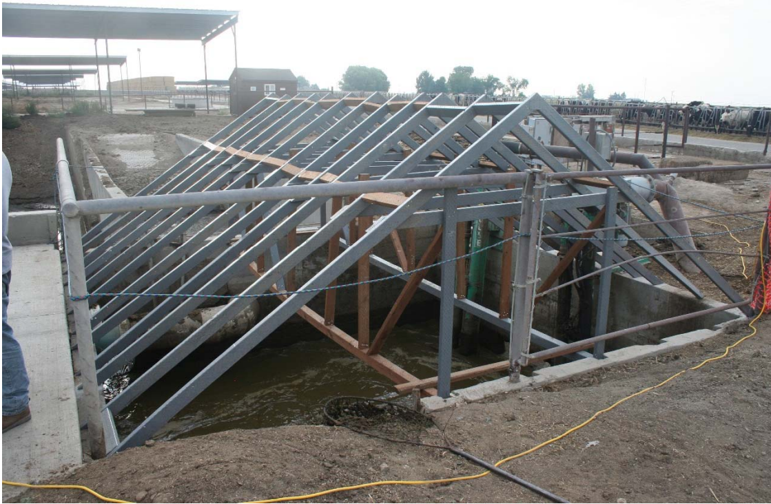
Picture 4. 17 Frame of the pit covering structure
