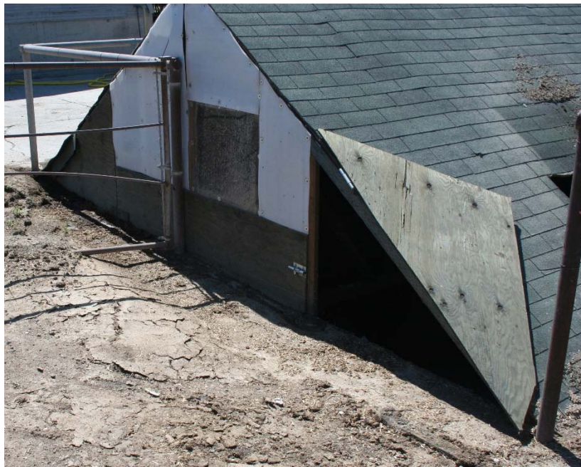
Picture 3. 4 Detail of maintenance access door
