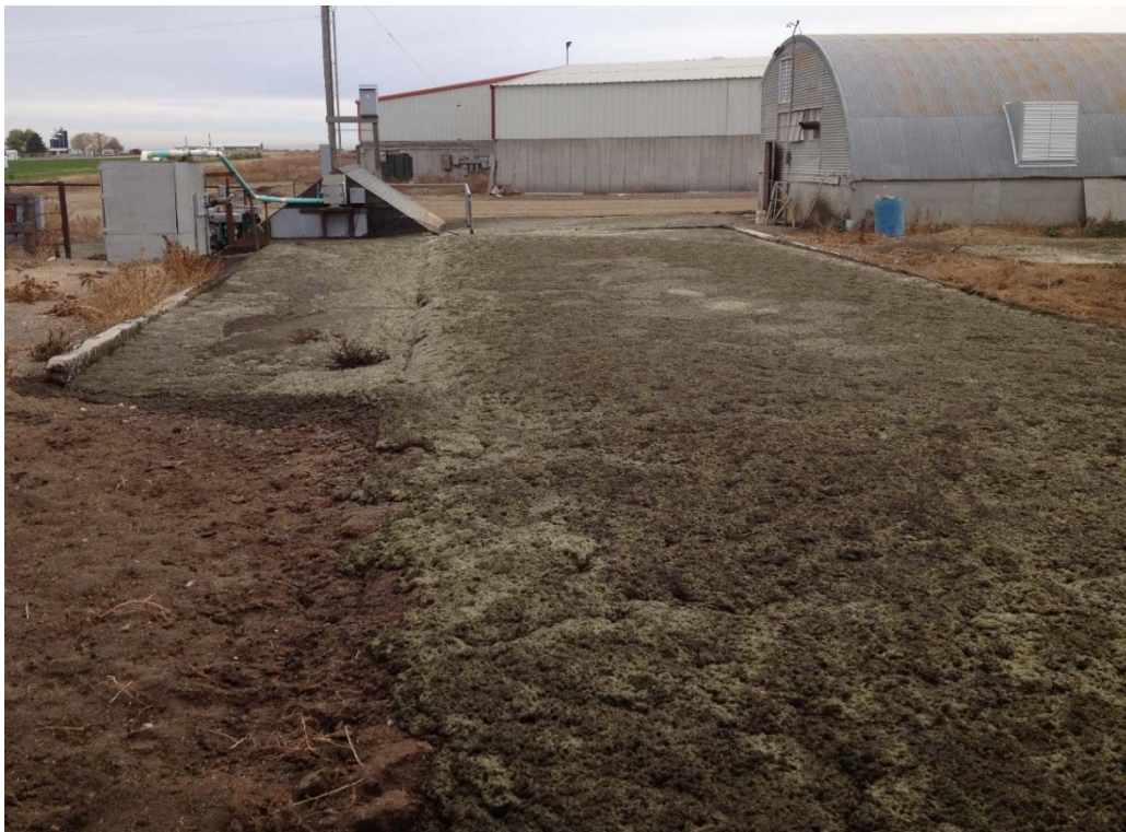
Picture 3. 14 Gravity separators totally covered by foam
