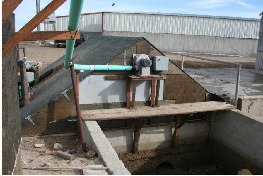
Picture 4. 21 View of back of the pit cover structure
