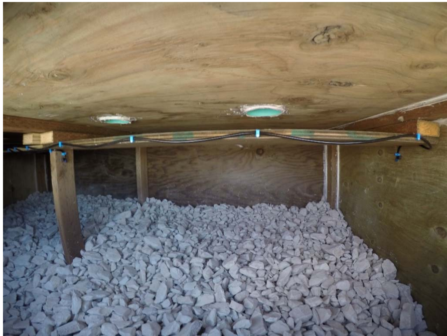
Picture 4. 8 Internal view of inlet, diffuser and watering sprinklers
