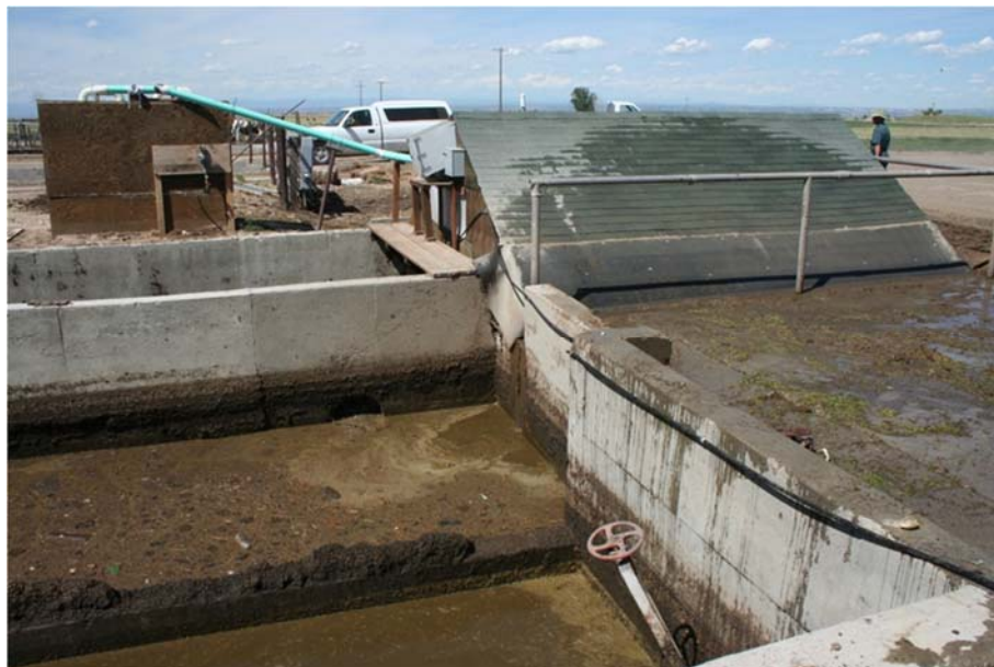
Picture 4. 20 Side view of cover structure, back of filter, and washing pad
