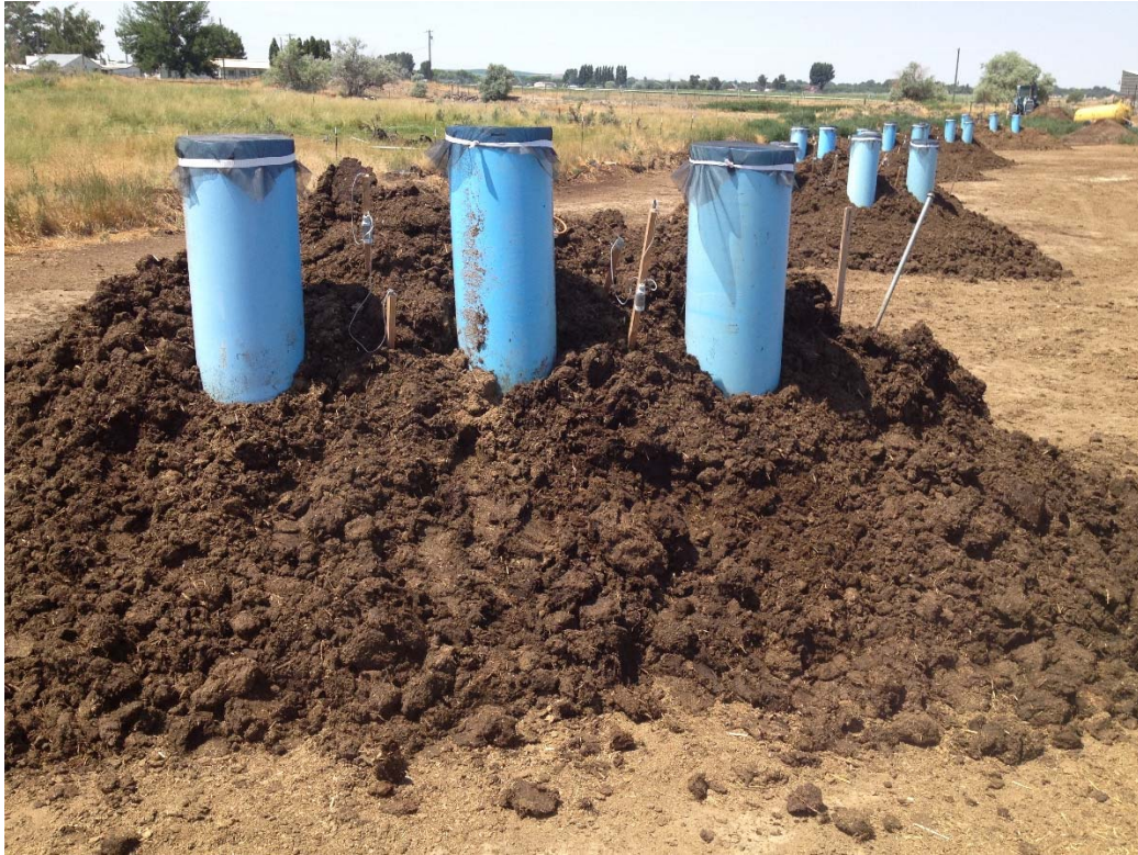
Figure 2. 9 Pipe “chimneys” resting on top of compost
