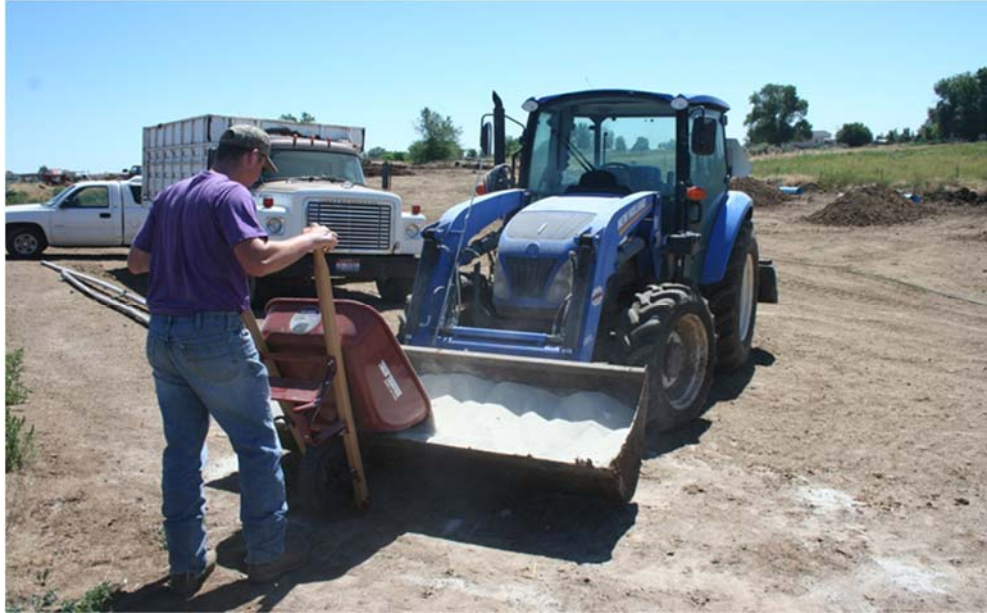
Picture 2. 5 Preparing for clinoptilolite addition to recipe
