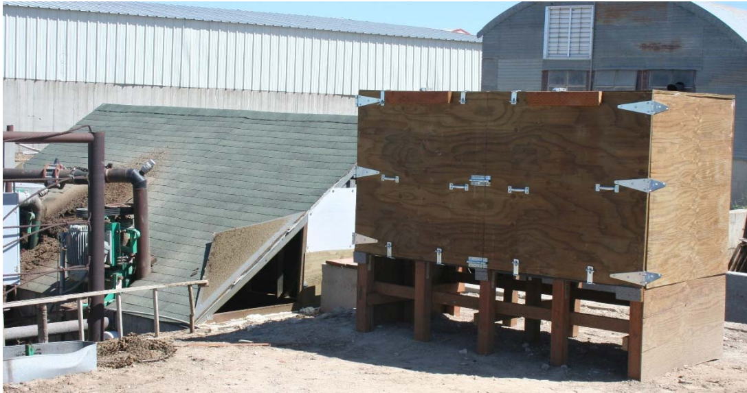
Picture 4. 3 Filter top section full enclosure and doors with locking hardware
