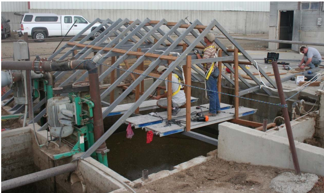
Picture 3. 2 Building the frame of the pit covering structure
