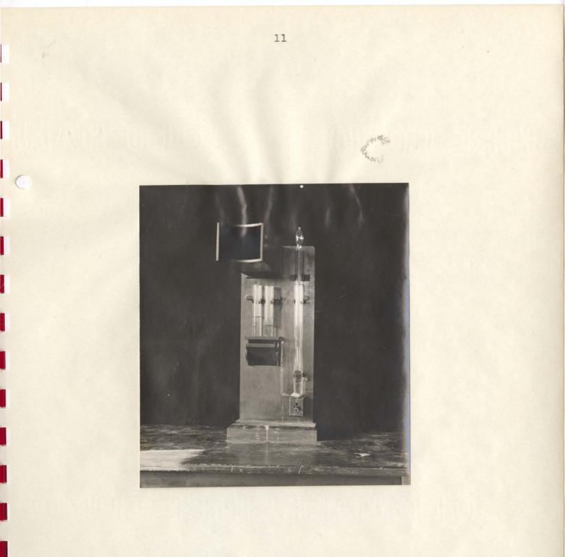
Plate I. Colorimeter used in making the tests for nitrites and nitrates.
