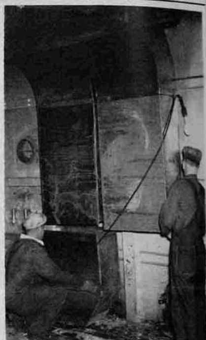
Above—Wm. Briere and Fay Berry at work on the installation of forced draft apparatus for the furnaces at Clearwater. Hot air will be taken from underneath the boiler deck and forced over the top of the fire in the furnace fire box. In that the air will have been pre-heated, better combustion with less discharge of cinders out the smokestacks is expected.
