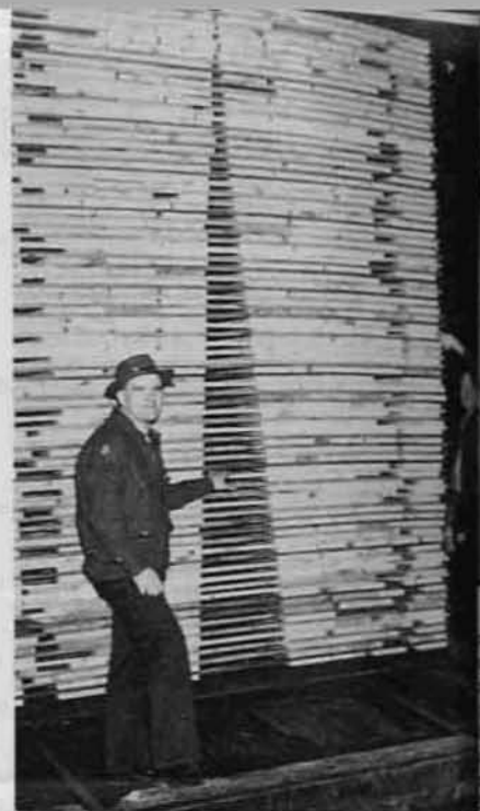
Above—Clearwater kiln foreman Phil Reinmuth and veteran kiln man Henry Steffelback. An experienced kiln man like Steffelback can tell how dry lumber is by one quick swipe of the handle of his pocket-knife down the side of a load.
