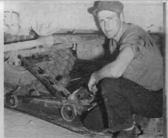
Above—Harris Mithoug, Camp 40 mechanic, designer of a time and labor saving apparatus to aid the removal of logging truck rear ends, transmissions, etc.
