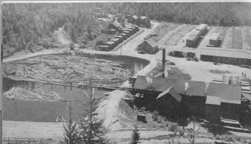
Above—Lewis mill, purchased by P.F.I. in July. Mill is located about eight miles from Bovill along road to Camp 46, Badger Meadows, employs around 60 men. It was in good shape, with excellent housekeeping.
