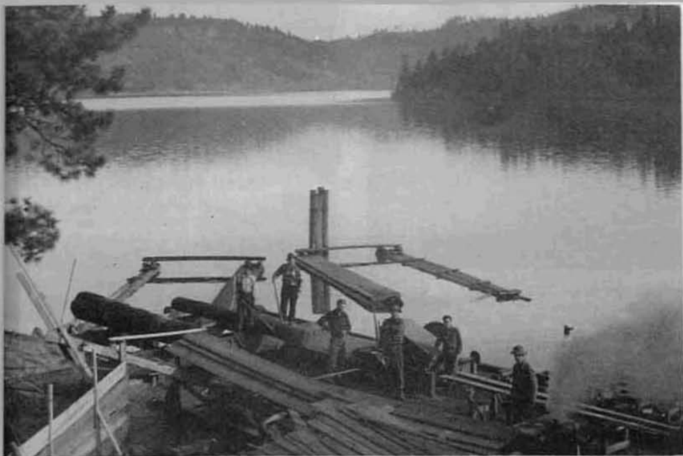
The mill at Squaw Bay . . . a six-man crew against a background of lake, forest and sky. The addition of an edger and trimmer will increase output. Roof will be added later for protection against the weather. Note U-shaped rafts which are used to transport salvaged logs.
