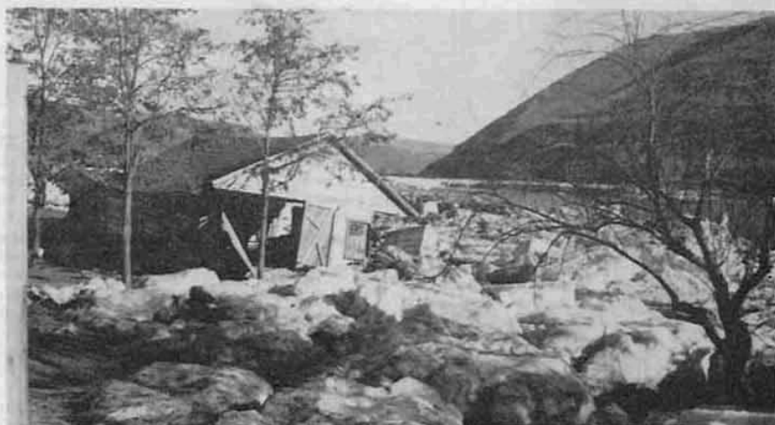
ICE JAM —Late January brought a strong chinook wind and a quick break-up of ice in the Clearwater. Despite quick action at the Washington Water Power dam (Lewiston) it was impossible to prevent pile-up of ice along the river from Lewiston to Spalding. This building, well above ordinary river level at high water, happened to be in the path of the moving jam. The resulting havoc is sufficient tribute to the weight of a moving ice pack.
