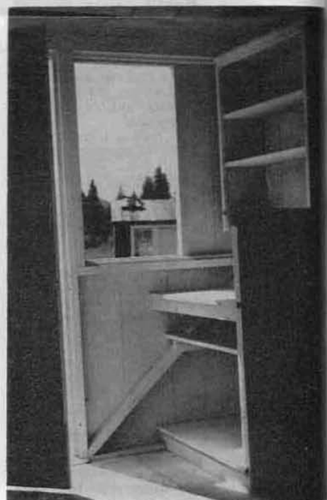
At left of entrance inside house are built-in cupboards for convenience of housewife. Beyond cupboards is space for stove where wall area is protected against heat by tacking sheets of tin to studding.
