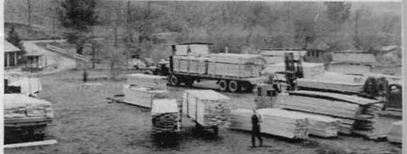
Loading out trucks at Clearwater.
