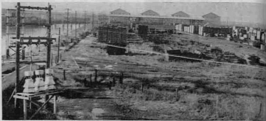
Above—Site north of tailrace where veneer plant will be located.
