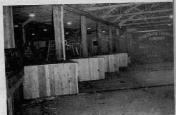
Right— Sawtooth dock eliminates much jockeying of truck and trailers into loading position.
