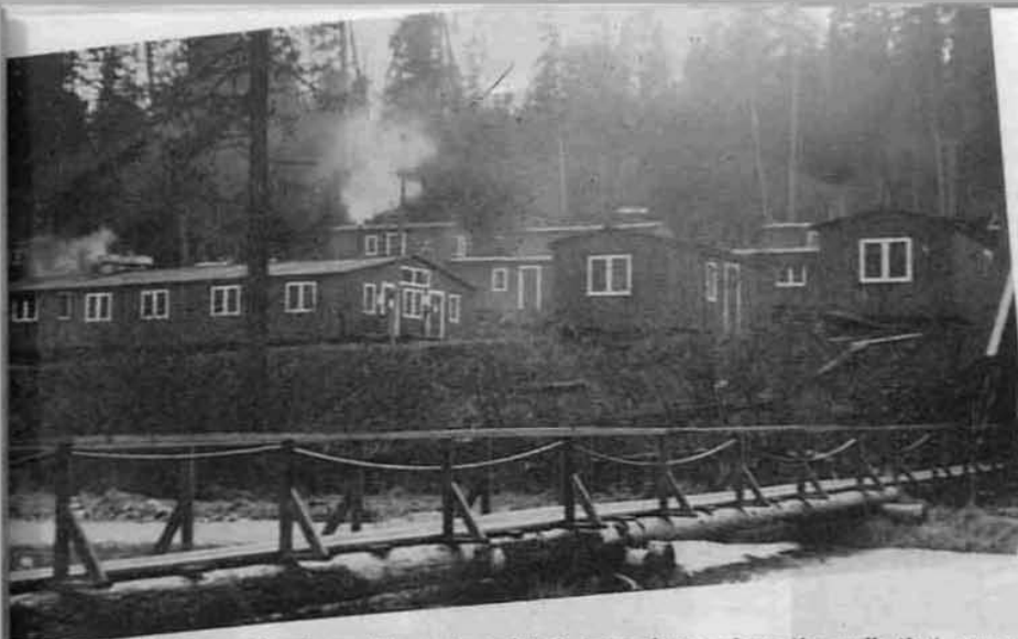
Camp 58, McComas Meadows. The main cable is here strung along the walk that crosses Meadow Creek spanning the distance between power house and main camp buildings.
