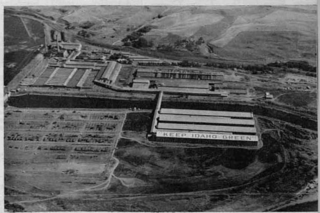
TWENTY YEARS YOUNG —Across the roof of the north rough shed at Clearwater has been painted words of advice that need frequent repeating . . . "Keep Idaho Green." Work was performed by sign painter Sam Canner and one helper and began of a morning at 4 A.M., continuing until around 10 A.M. when roof temperatures became so high as to set fire to a painter's feet. Letters are 32 feet high, 34 feet wide. The perpendicular strokes are eight feet wide, the horizontal are six feet wide and an average of two gallons of paint per letter was required for one coat. The building is 810 feet long, spacing between words and at ends is 38 feet, and there is six feet of space between bottoms and tops of letters and edge of roof. The two painters were able to average a letter per day, each.
