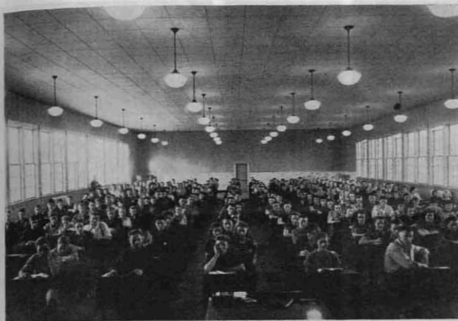
Built last summer, this huge assembly room of the Potlatch high school seats several hundred young men and women during the study hour. The walls here are of knotty pine wainscoting, Nu-wood plank and genuine Idaho white pine window frames and sash. There are 32 windows in the room. The ceiling is of Nu-wood tile.
